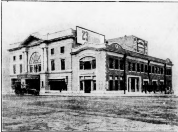
Located in Lawrence, Kan., the Bowersock is one of the modern theaters in the Middle West. It is thoroughly fireproof. Only the best class of road attractions are shown, motion pictures filling open dates.
